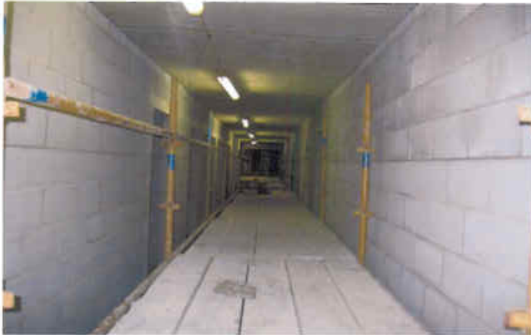
Photo 9: Basement -2 Blockwork – Circulation Corridor (as at 8/9/10)
