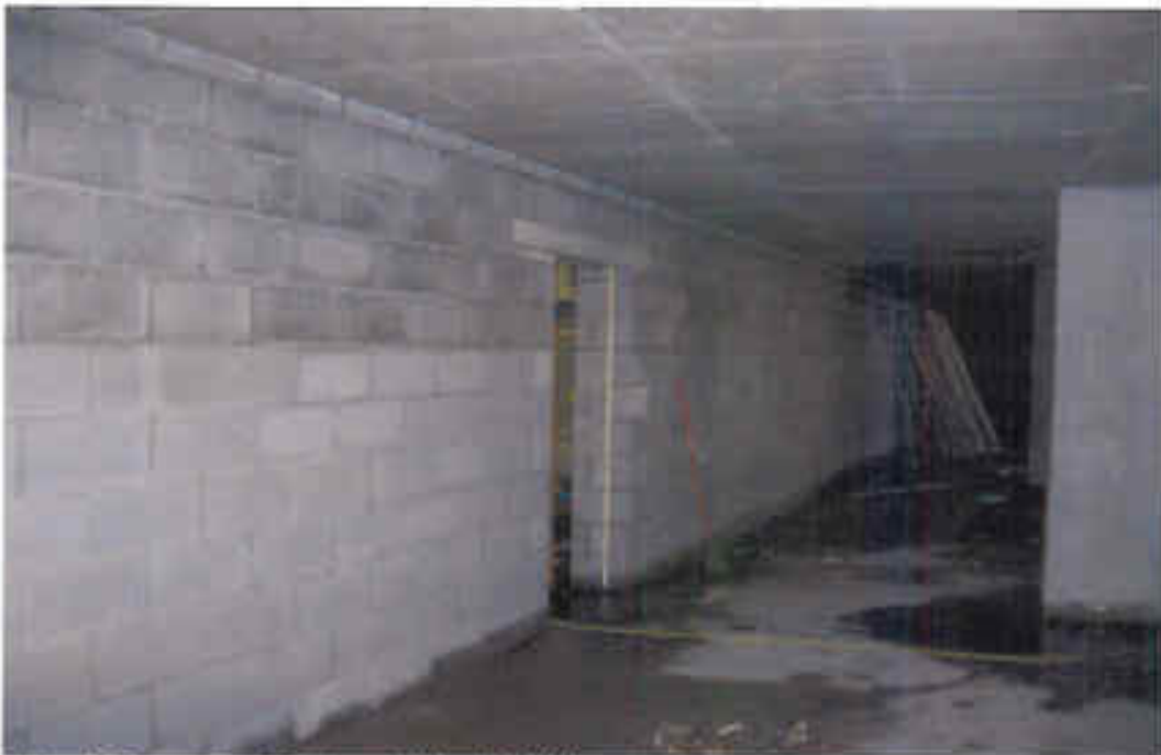
Photo 10: Basement – 2 Blockwork: (As at 8/9/10)
