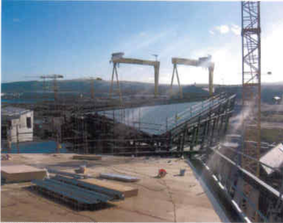
Photo 15 Hull 4 Roof (as at 30/9/10)
