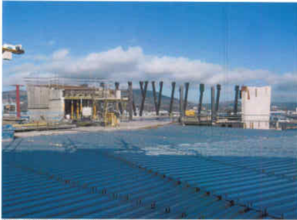
Photo 17 Roof view over Hull 1
