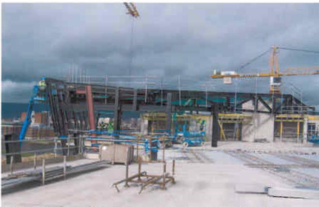
Photo 4: Hull 4 Roof Steel (Note: MBF in cherry picker working on cladding rails) (as at 8/9/10)
