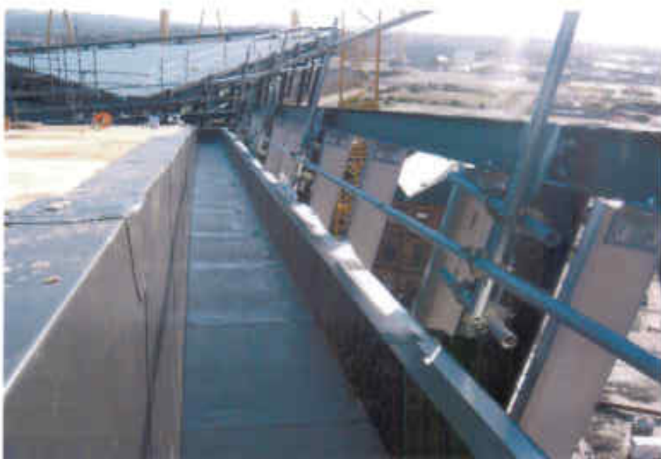
Photo 14 Hull 4 roof guttering (as at 30/9/10)
