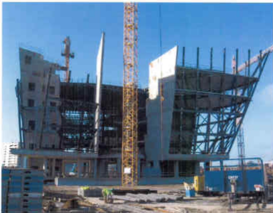
Photo 18 North Elevation (As at 30.09.10)
