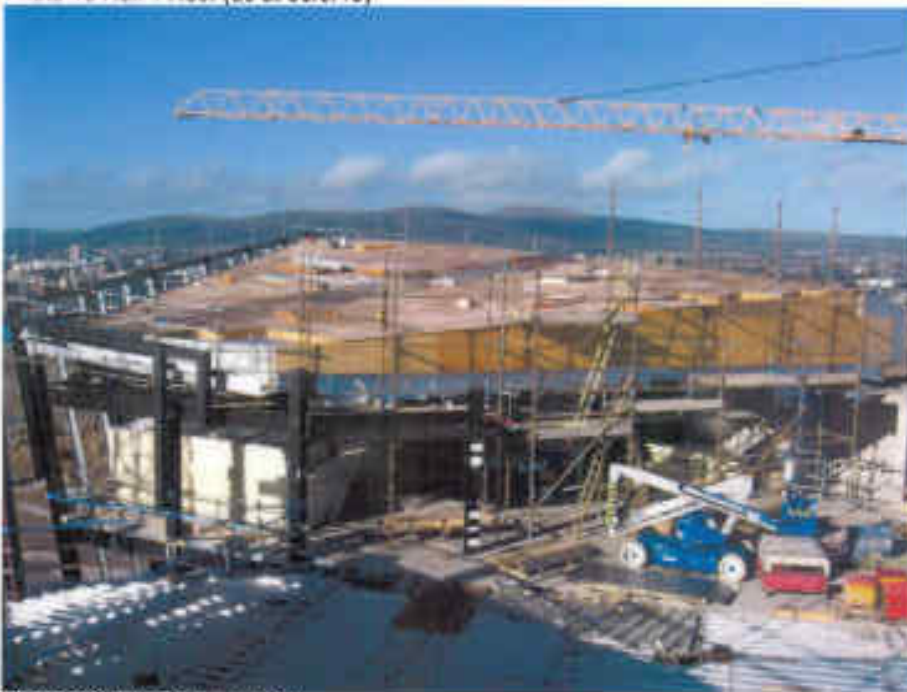
Photo 16 View of Hull 4 Roof
