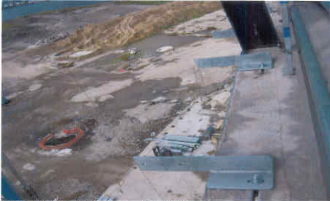
Photo 5: Hull 4 Cladding Rail Brackets – Level 5 (as at 8/9/10)
