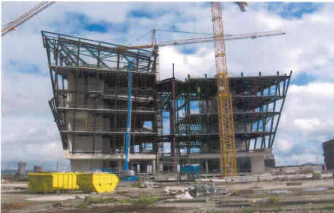
Photo 2: View of South Elevation (as at 8/9/10)
