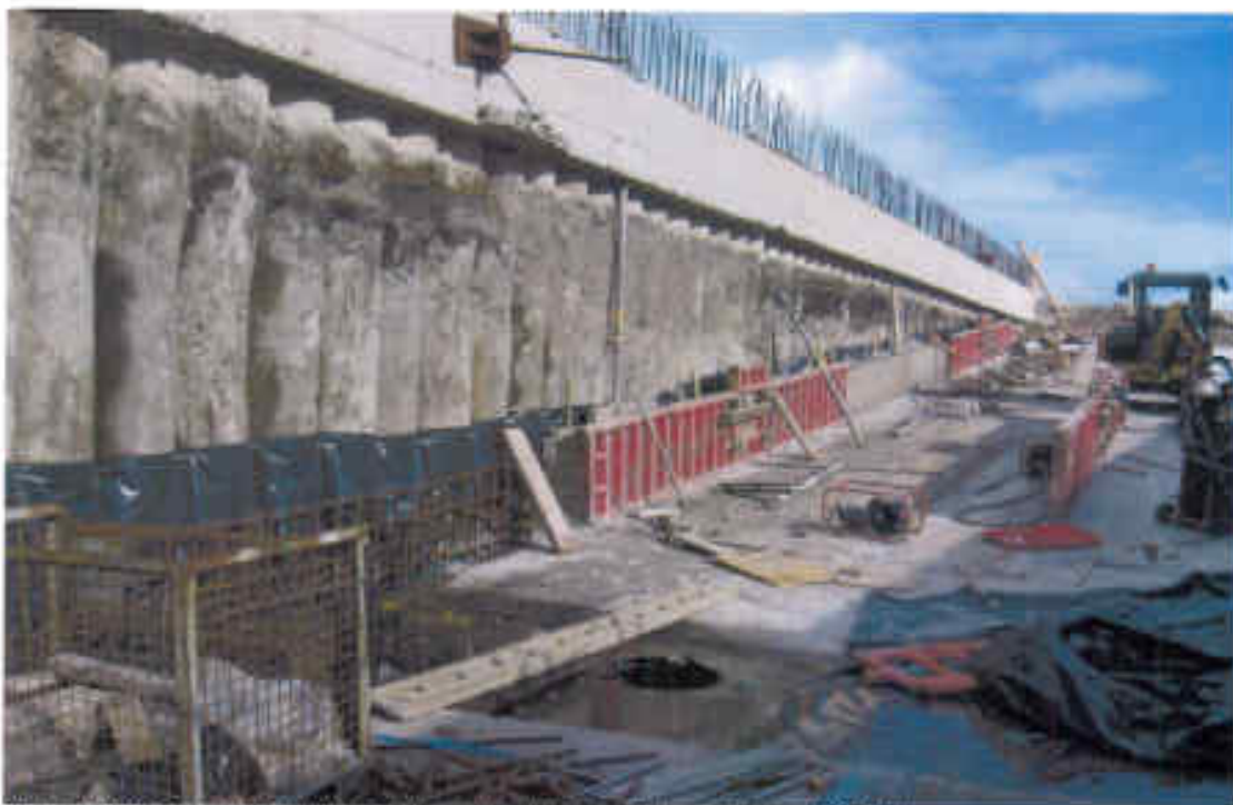
Photo 8: NW Service Yard Ramp with up-stand wall partially cast. (As at 8/9/10)
